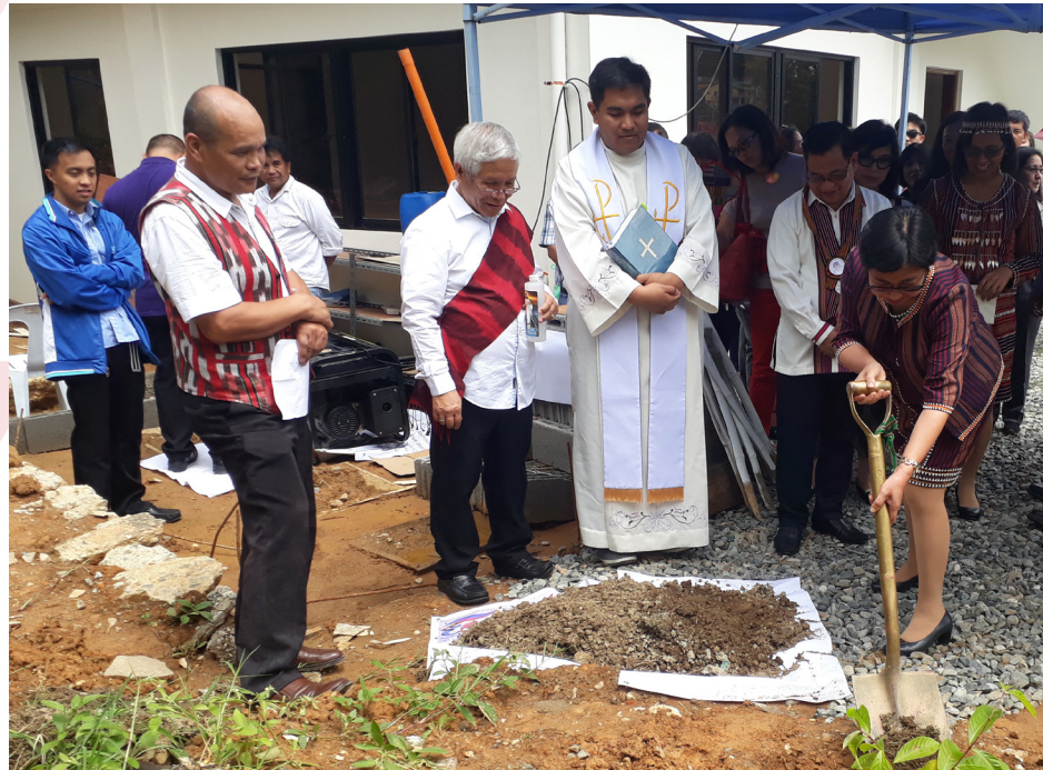
CSC Regional Office CAR Director IV Marilyn E. Taldo (leftmost) leads the blessing and groundbreaking ceremony of the CSC Field Office in Benguet.
